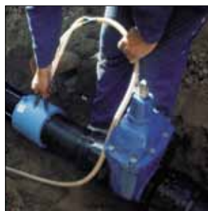
Socket fusion welding is a fast and effective technique
