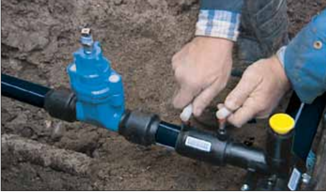
Installation of a service connection valve with PE-ends
