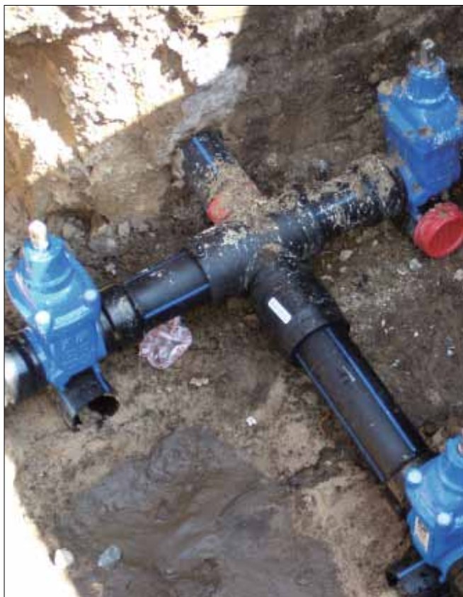
Installation of a PE-pipeline
