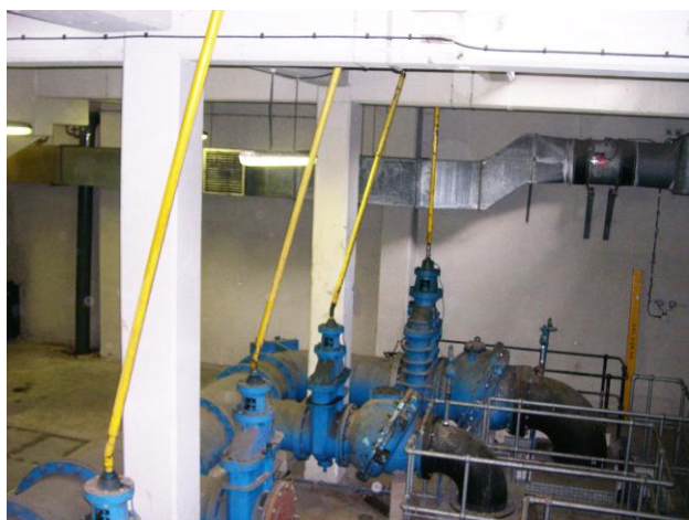
Photograph 1 Original Main Pumping Station
