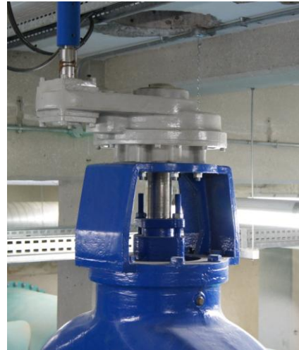
Photograph 7 AVK Series 54 Geared Gate Valve
