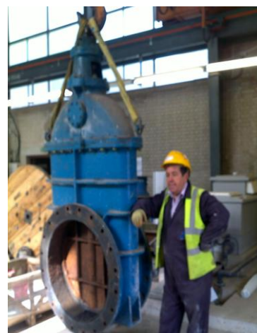
Photograph 2 Removed DN800 Original Valve
