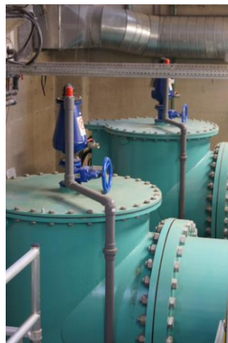
Photograph 9 Series 701 Waste Water Double Acting Air Relief Valves With Piped outlets
