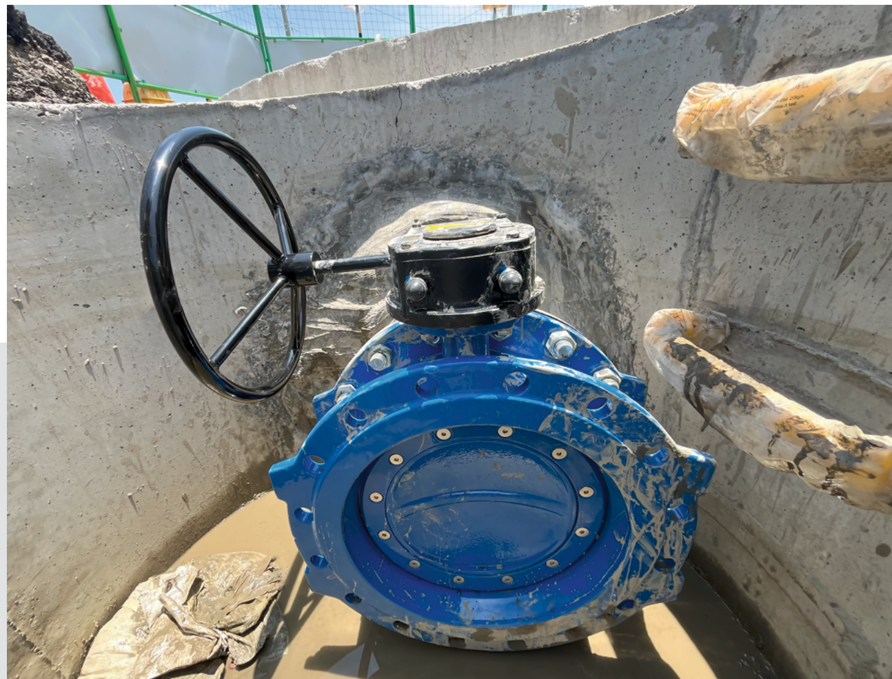
Butterfly valve installed
